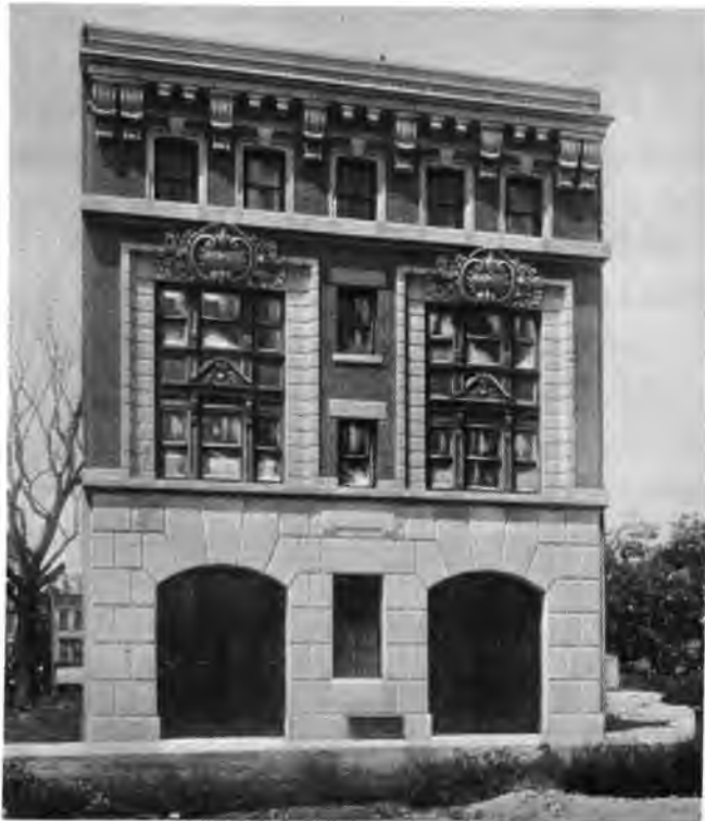
EXTERIOR OF SUB-STATION NO. 18
